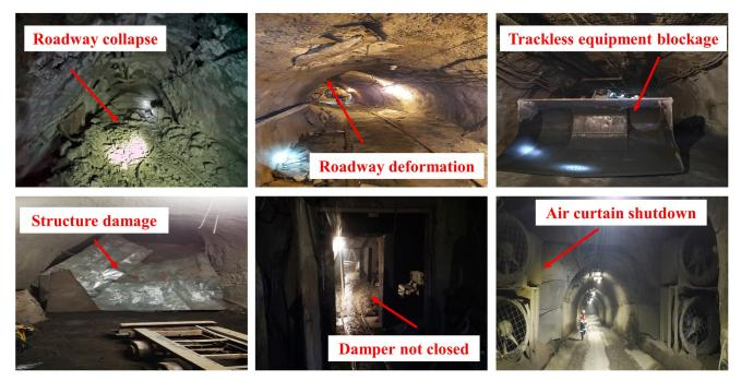
Fig 1. Resistance variant faults in a real mine. (Created by the author).
