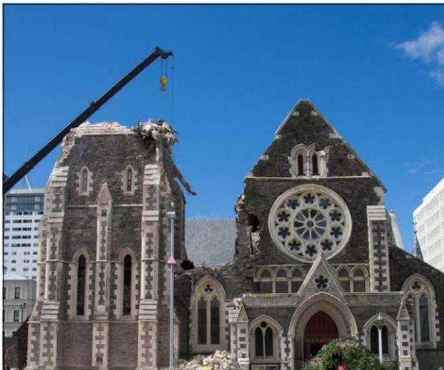
**Figure 1. The top figure shows the Christchurch National Anglican Cathedral, a city landmark, before the 22 February 2011 earthquake. The bottom the figure shows the Cathedral after the earthquake. Images were taken from Wikipedia Commons subject to the GNU Free Documentation License.**
