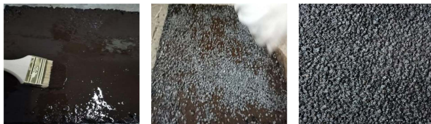
(a) Brushing emulsified asphalt (b) Spreading aggregates (c) Spraying sand-containing fog seal
