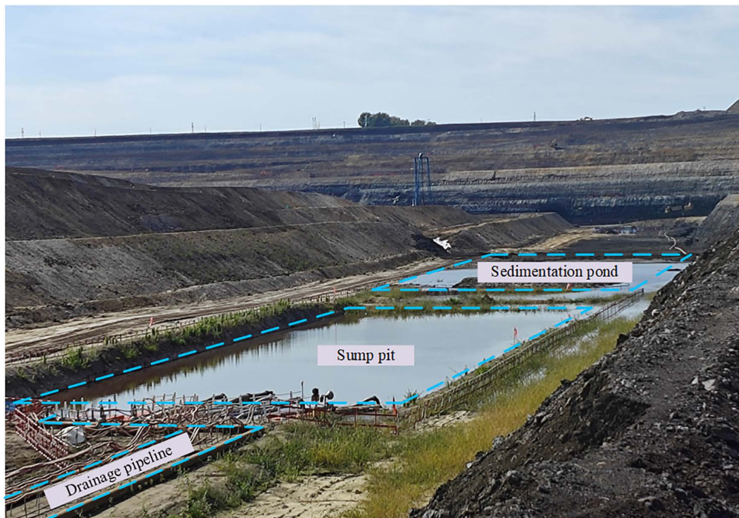
Fig 15. Field sump, sedimentation pond, and drainage pipeline. The photograph was taken and annotated by the authors.
