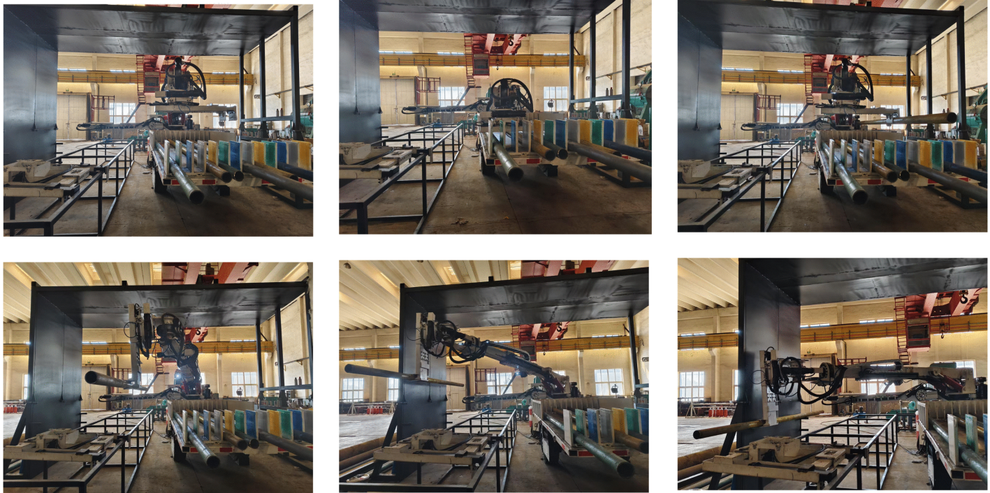
Fig 19. Actual movement process of pipeline installation robot. (a) a_1 point; (b) c_1 point and c_2 point; (c) a_2 point; (d) f point; (e) d point; (f) e point.
