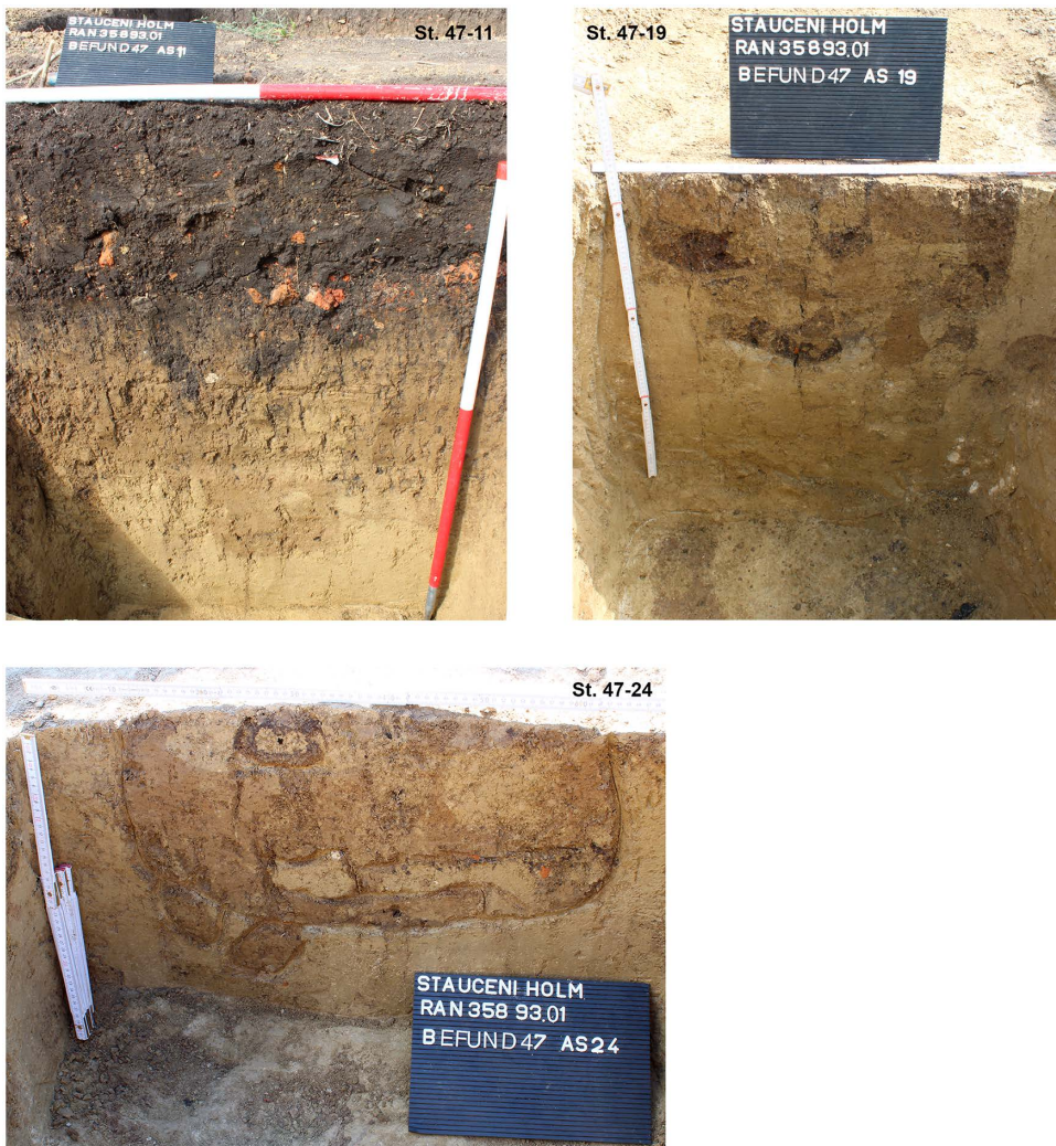
Fig 21. Stăuceni-Holm'. Mega-structure house 5/6. Sections through the foundation ditch and the postholes No. 47-11, 47-19 and 47-24 within the ditch. For the location of the sections see Fig 19 . All used pictures made by the author (C. Mischka): – three photographs of excavation profiles.
