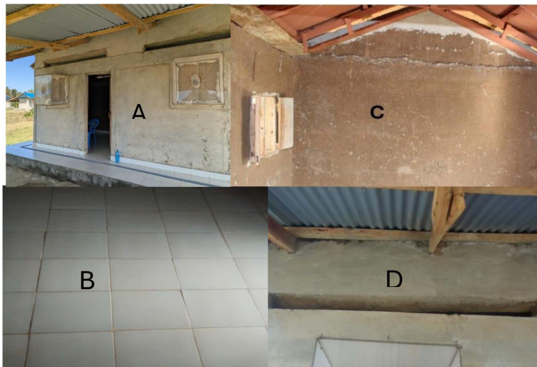
Fig 1. Experimental hut design: A front view of the hut fitted with window exit traps, B showing the tiled floor and the hut interior walls C showing the wood baffles and D showing eaves.
