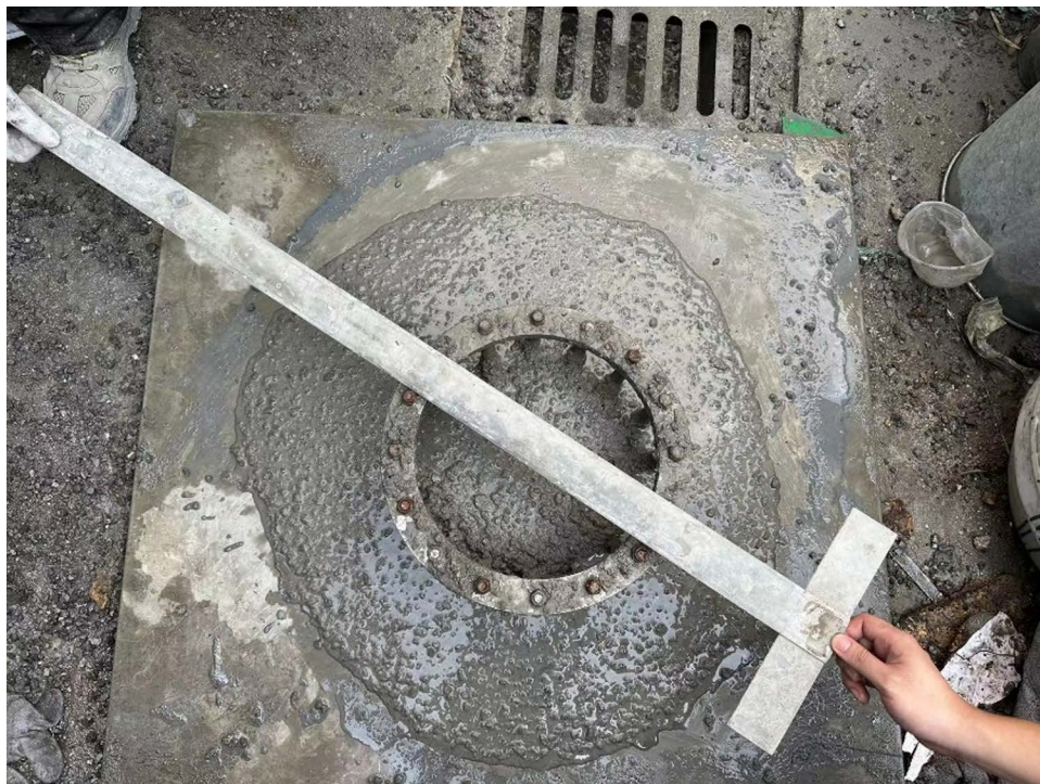
Fig 3. J-ring expansion of steel fiber self-compacting concrete.
