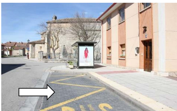
Fig 8. Protection at bus stops. Road markings indicating bus stop.
