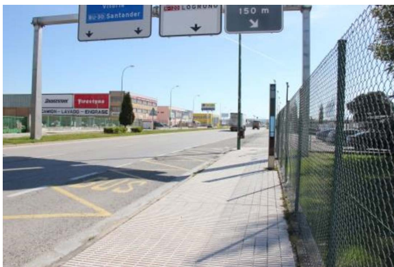
Fig 6. Bus stop with step-free access located over 100 metres away.
