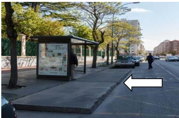
Fig 7. Protection at bus stops. Platform extending from the sidewalk.
