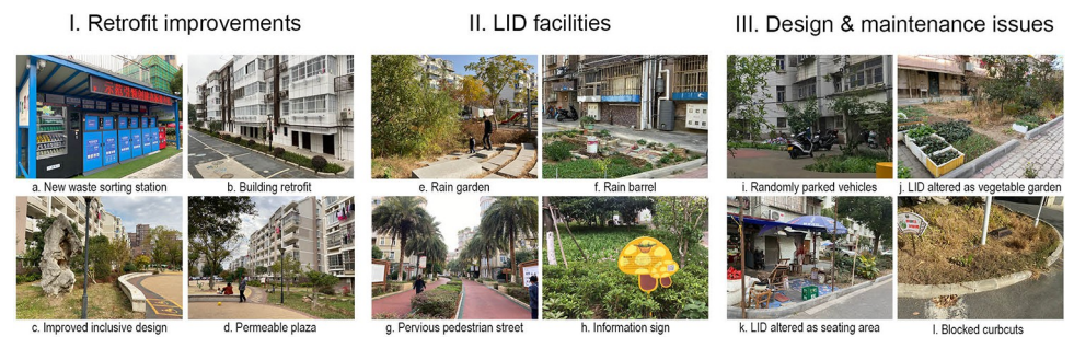
Fig 5. Examples of retrofit improvements, LID facilities, and design and maintenance issues. All photos by Authors 1 and 2.
