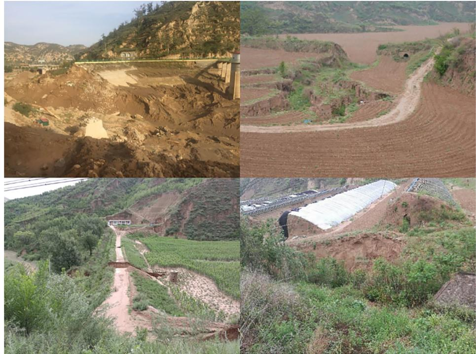
**Fig 2. Breach of check dams in Suide County.**
