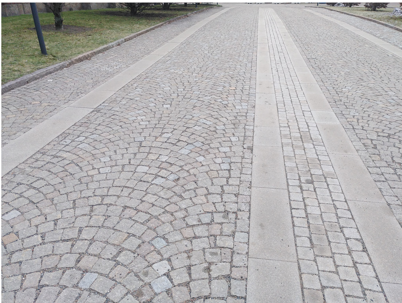
Fig 2. Cobblestone road surface for outdoor tests. The tests were carried out between the concrete slabs.
