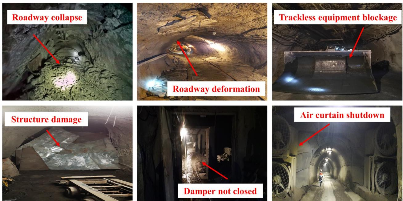
**Fig 1. Resistance variant faults in a real mine.** (Created by the author).
