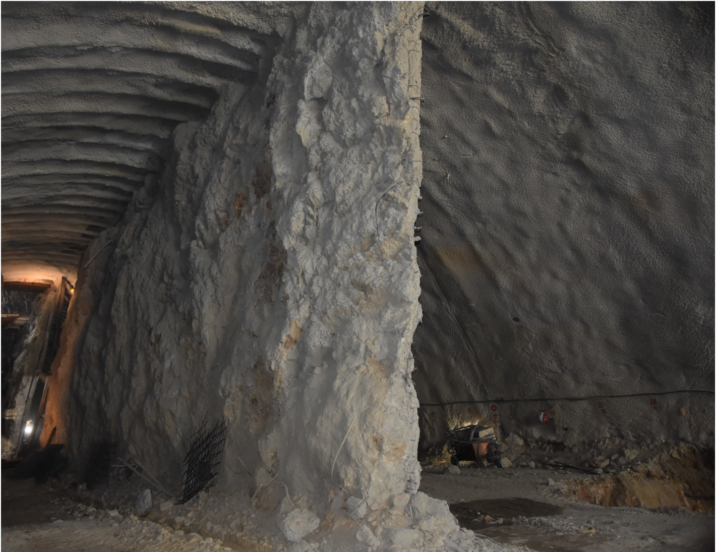
Fig 2. The construction of middle wall structure.
