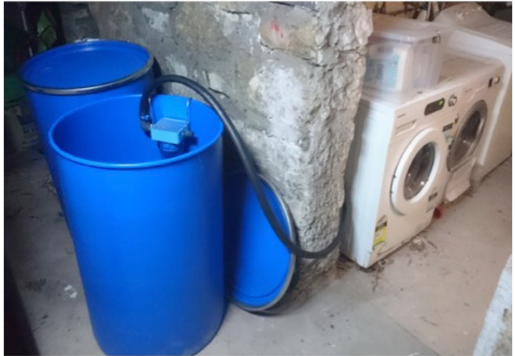
Fig 2. Filters connected to domestic appliance and 200 L polyethylene drum.
