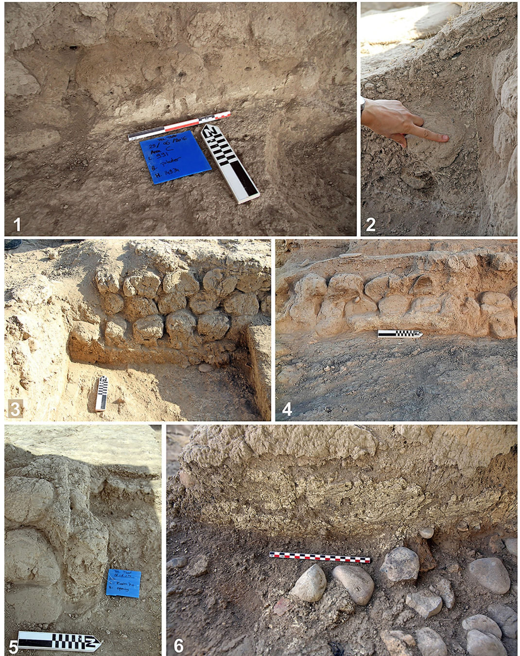
Fig 8. Examples of the plaster coatings of the interior walls of Room C70 and exterior wall of Structure 286. Note the variety of thicknesses.
