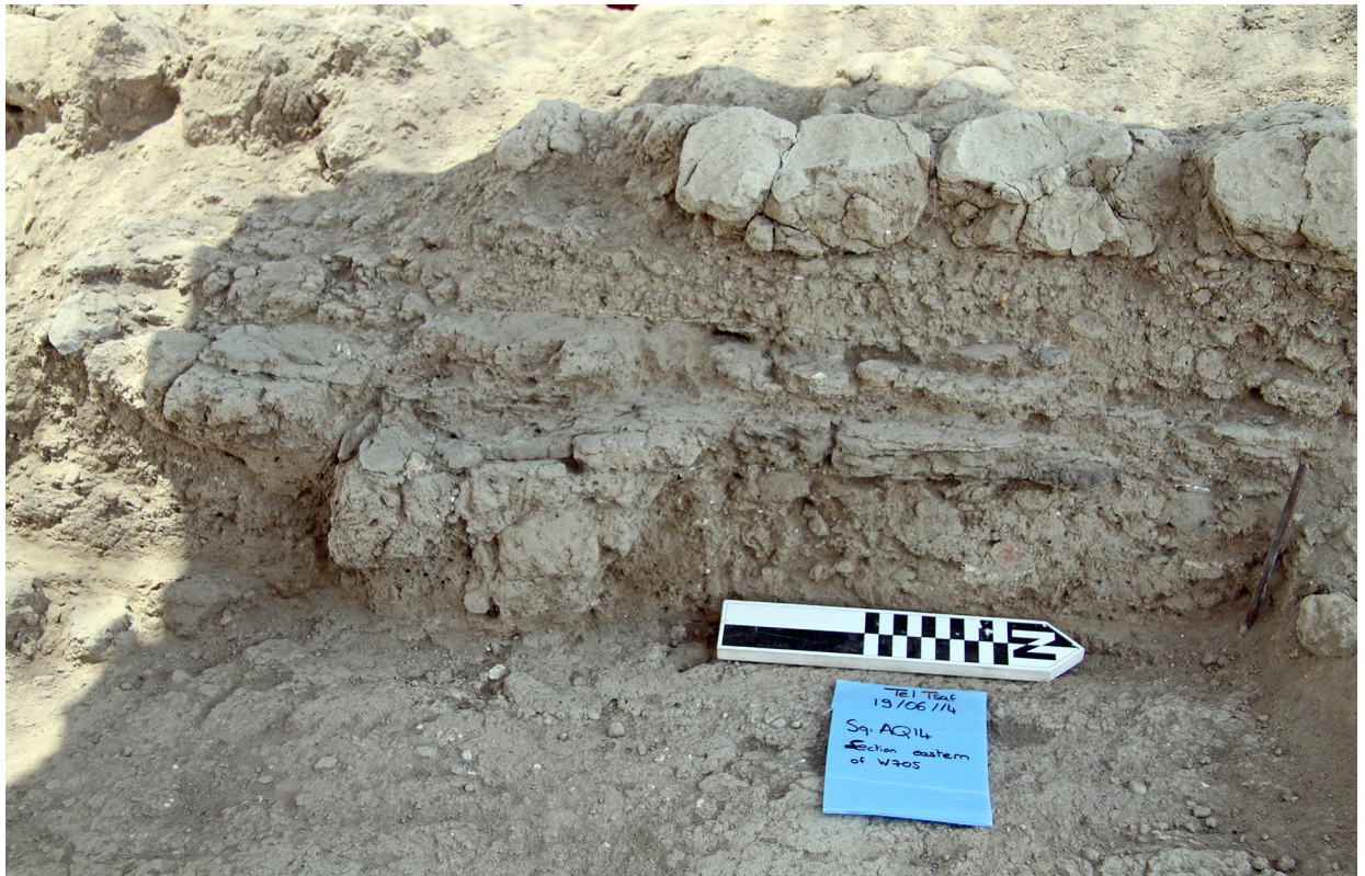
Fig 7. Plastered floor levels in the section of Room C70.
