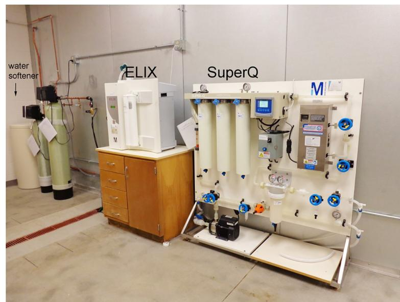
**Fig 1. Components of the system that produces ultrapure water.**
