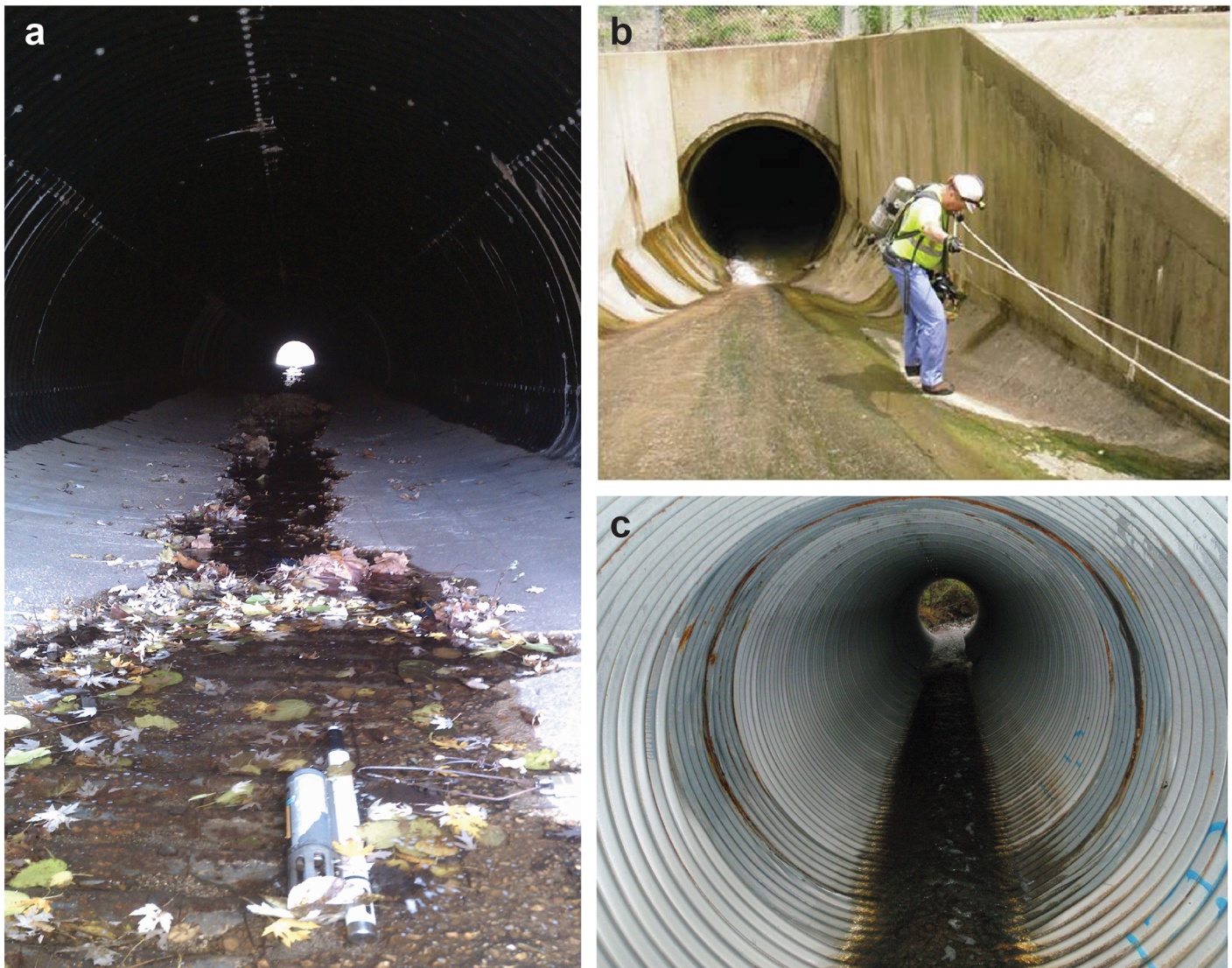
Fig 1. Stream burial is an extreme, but ubiquitous, consequence of urbanization in stream ecosystems. The buried stream channels in the cited studies were constructed from various materials including (a) a cement-lined corrugated metal pipe in Baltimore, Maryland (USA), (b) a concrete tunnel in Cincinnati, Ohio (USA), and (c) a corrugated metal pipe in Cincinnati.
