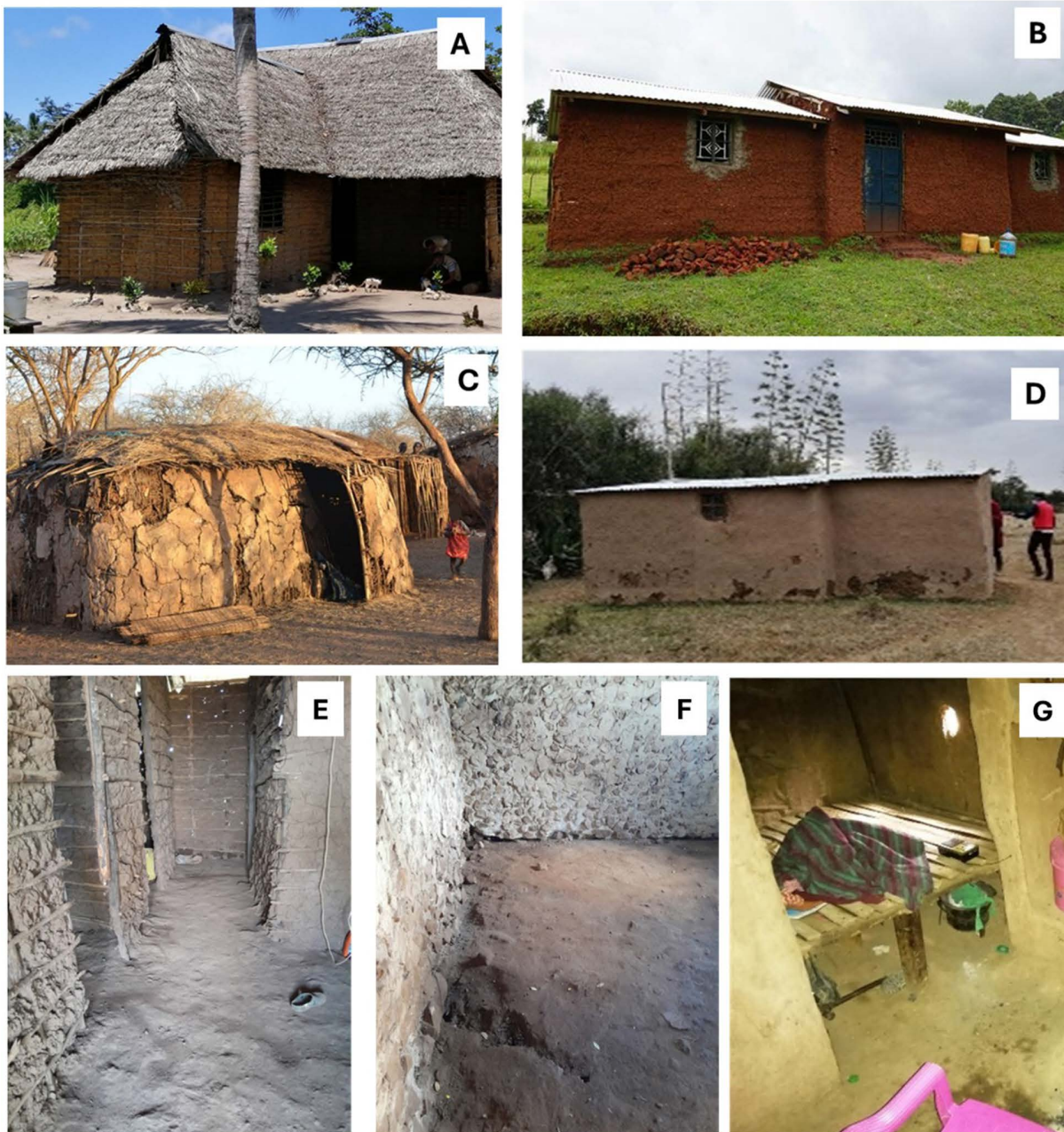
Fig 2. Traditional house structures and floors. Building in Kwale (A); building in Bungoma (B); traditional Maasai house and (C) modernised Maasai house (D) in Narok. Typical unimproved earthen floors in houses in Kwale (E), Bungoma (F), and Narok (G).
