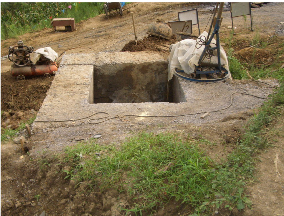
Fig 15. Anchor blocks at exits.
