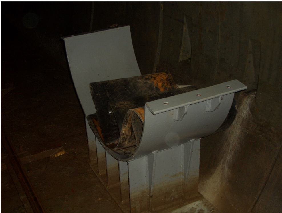
Fig 17. Steel sliding blocks.
