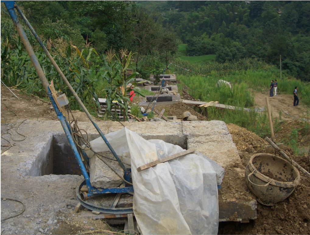
Fig 14. Anchor blocks at entrances.
