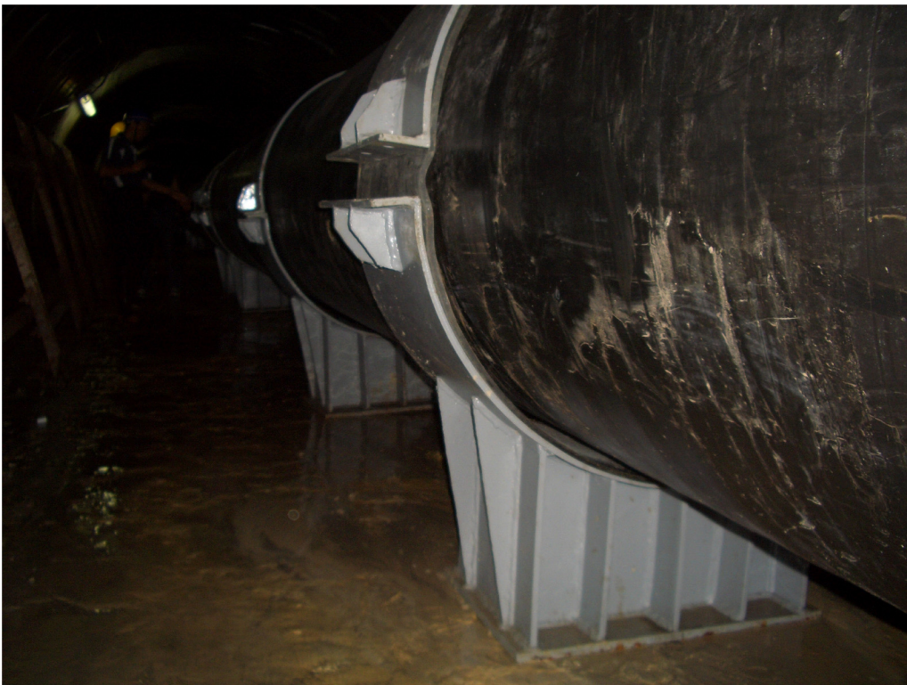
Fig 21. Unfixed pipelines.
