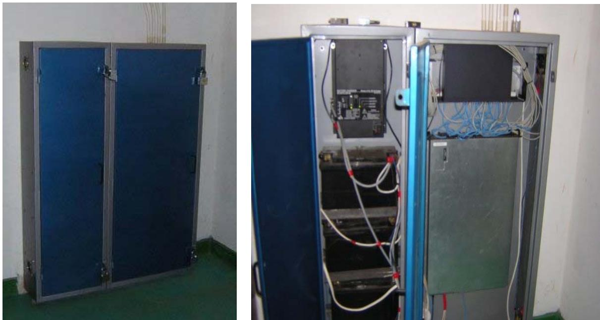
Figure S1.A: Battery backup cabinet collocated with server/network electronics cabinet
